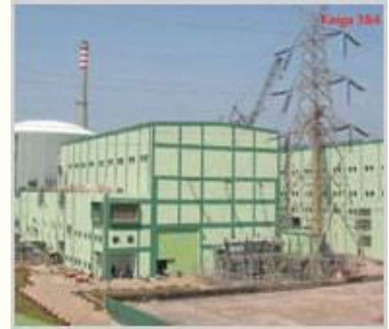
KAIGA ATOMIC POWER PROJECT
